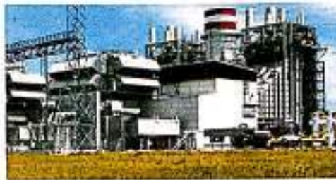
Venagiri Power Generation Limited. Proposed 370 MW Combined Cycle Power Plant at Andhra Pradesh
