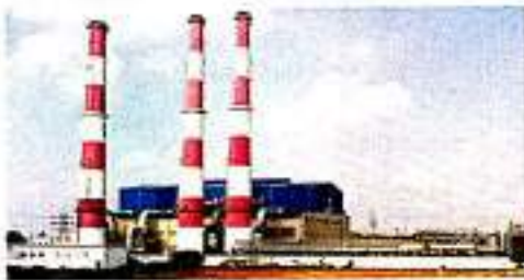
GMR Power Corporation Private Limited. The world's largest 2 stroke power plant at Chennai
